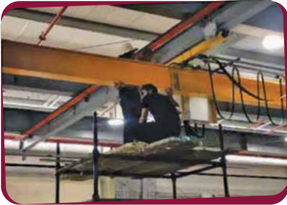
OH Crane Installation
