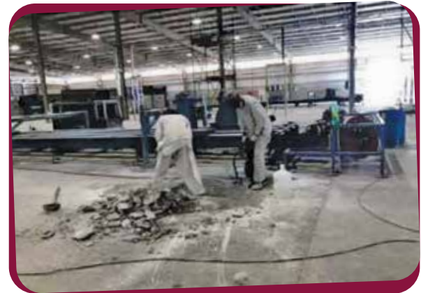
Concrete Floor Breaking
