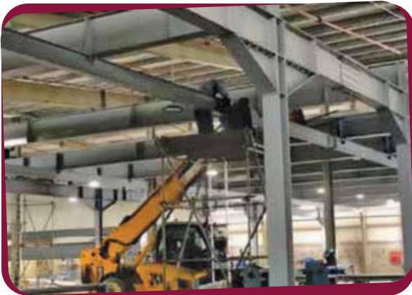
Crane Structure Erection
