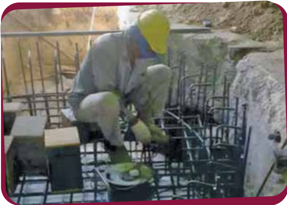
Re-Bar Installation
