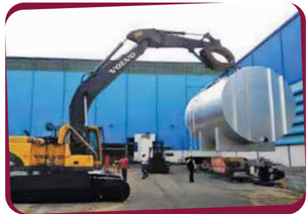
Diesel Tank Errection
