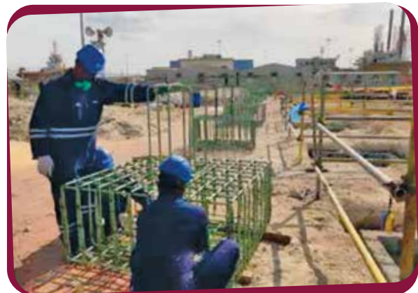
Foundation Rebar
